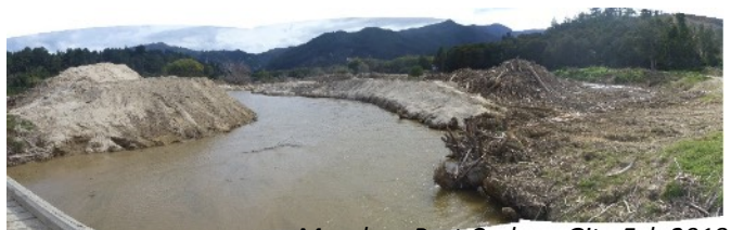
Marahau Post Cyclone Gita Feb 2018
